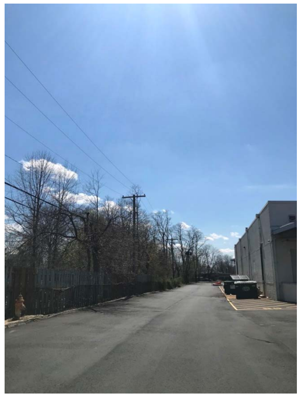
Photo 17 – Rear of building – east side
