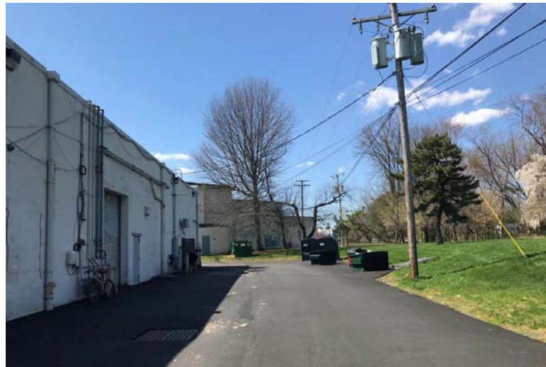
Photo 15 – Rear of building - north side
