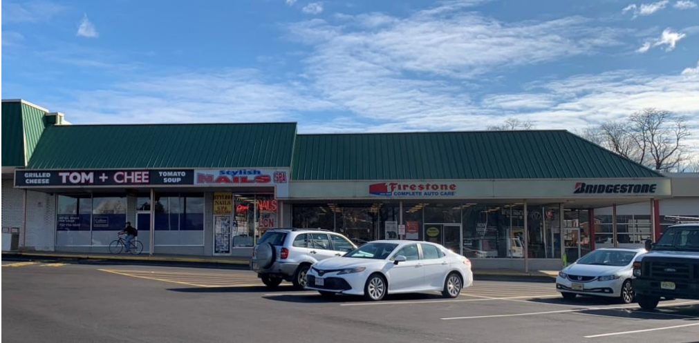
Photo 4 – Tom + Chee Restaurant (vacant) Firestone and Bridgestone Tire Store, Nail Salon
