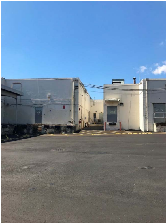
Photo 16 – Rear of building – east side
