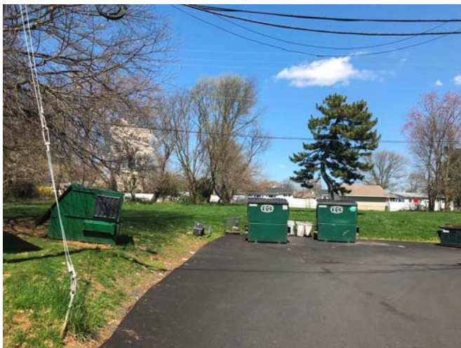
Photo 18 – Rear of building – north side
