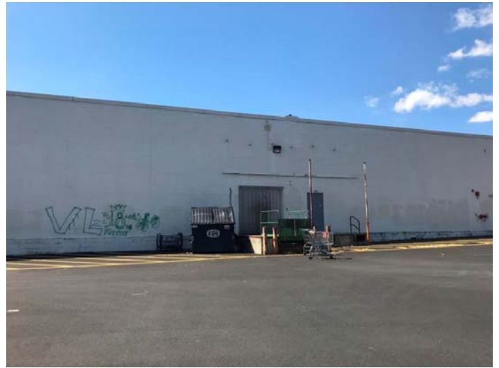
Photo 13 – Rear of building – east side behind Burlington Coat Factory
