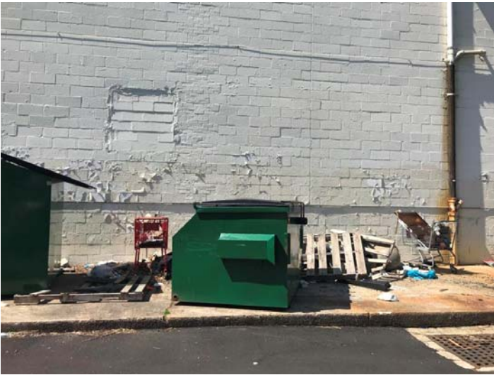
Photo 12 – Rear of building – east side
